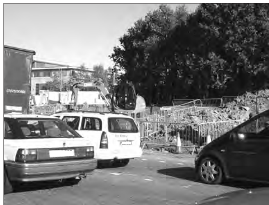
Under way: Work progresses at Segensworth.
