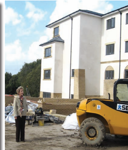
Visiting: Councillor Marian Ellerton looks at progress on the new building.
