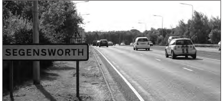
Wider: A fourth lane will be added to the link road from the M27 Junction 9 approach to the roundabout (above).
