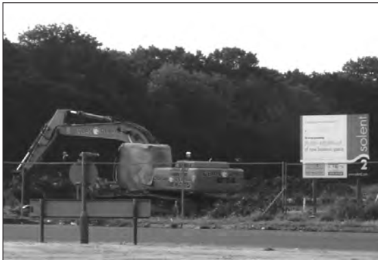
Ground breaker: A digger starts work at Solent 2.
